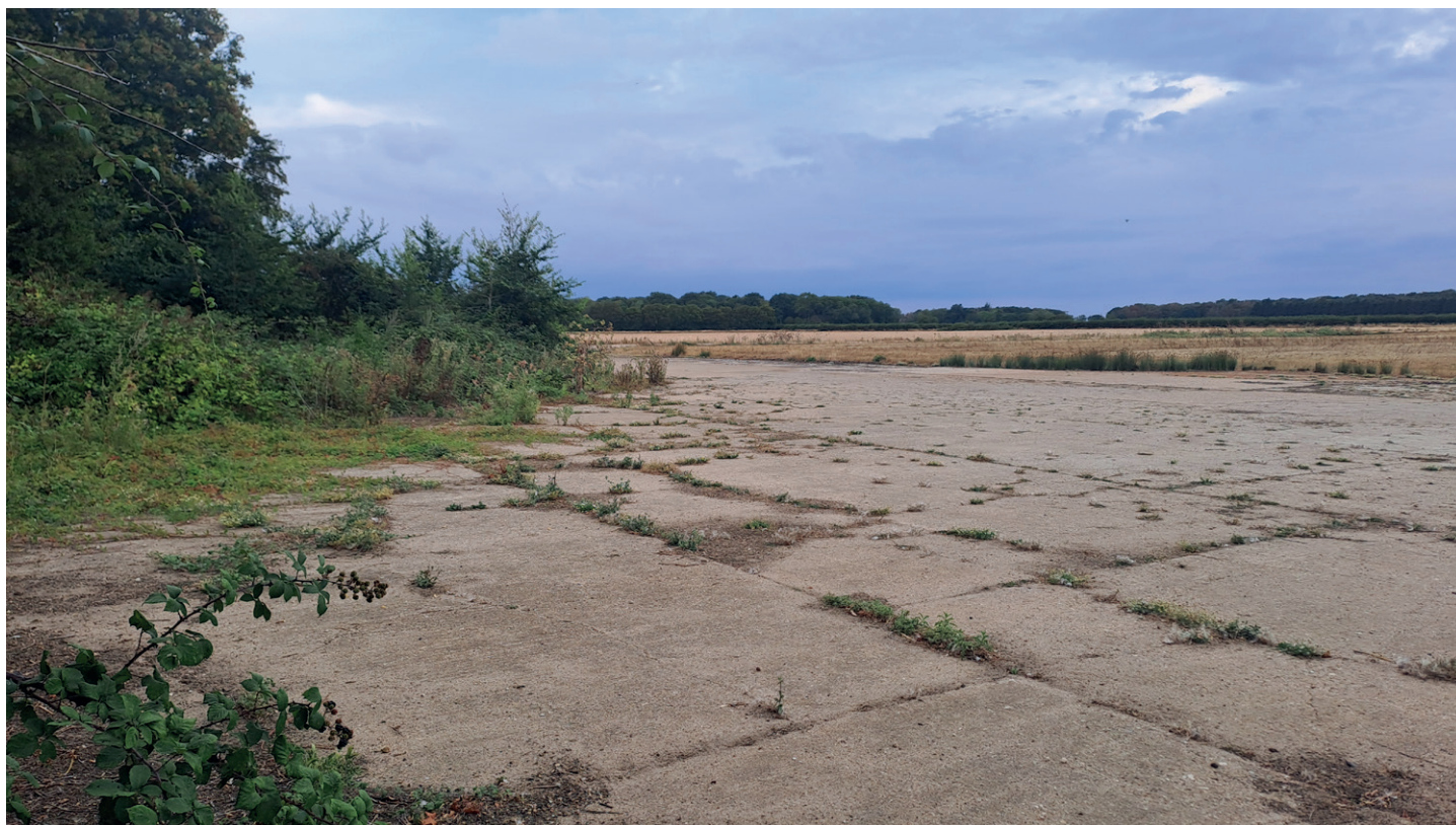
A today's look from Hardstand No. 5 to a section of the perimeter track.
